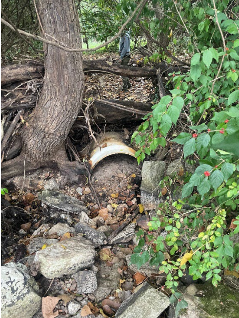
Photo 2 North side of crossing, facing north, close to road. Plugged pipe structure.
